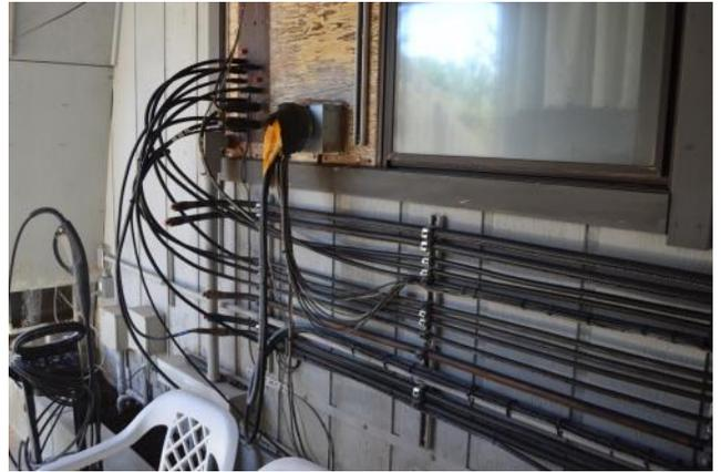
**Above:** Coax, including hardline, and control cables exiting the K6QXY operating position.
