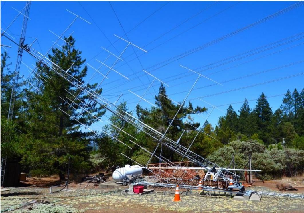
Lower: another view of the K6QXY EME array showing the tracks that move the base of the tower to change its elevation.
