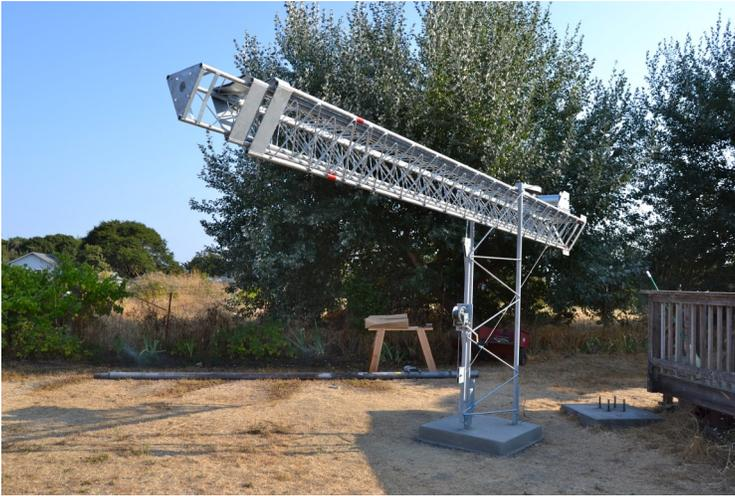
Top: the tiltable lower section of a Tasjian 52 foot tower during installation. Note that the top of the tower can be reached from a 10-foot step ladder.
